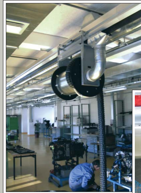
Mechanical hose reel, movable in rail system SSK 290.
