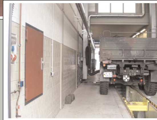
Rail system SSK 150 as travelling system at HGVs/LGVs brake test beds with single fan FD. Optional with automatic hose detachment from the exhaust and automatic return of the hose carriage via pulley drive.
